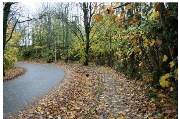
Existing pathway along Cheasty Boulevard
