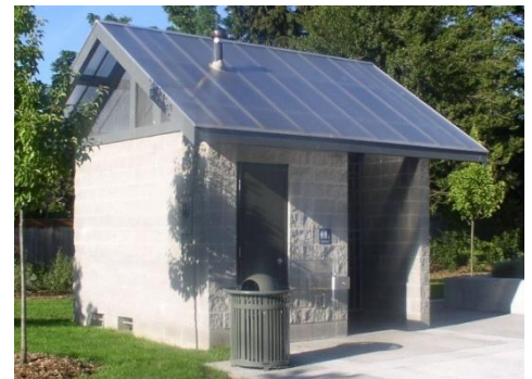
The new on-course restroom would be a unisex facility
