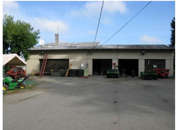
Existing maintenance facilities at Jefferson Park
