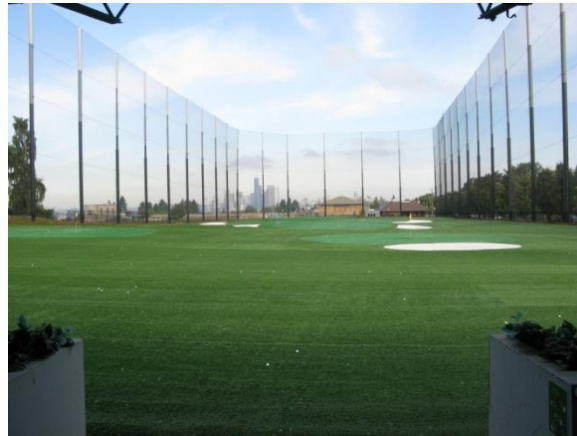
The existing single deck range shelter is in need of replacement
