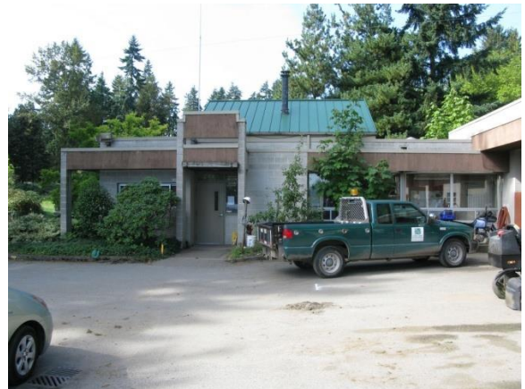
Maintenance facilities at Jackson Park require expansion.
